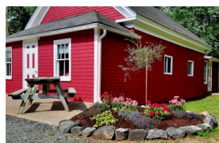
Upper Vaughan Community Hall
